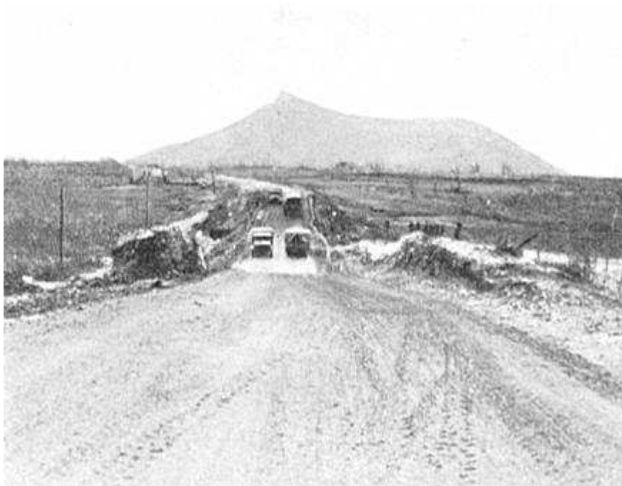
Figure 35. - Line 90. The railway track between Mignano and Cassino was removed and the formation used as a highway known as "Speedy Highway".
