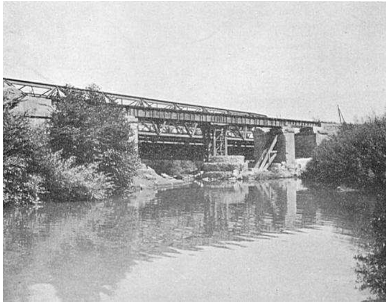
Figure 42. - Line 90. Bridge at Km. 65.867 between Sgurgola and Anagni. Reconstruction was carried out by 10 Railway Construction Company, R.E. from 8 June, 1944 to 28 June, 1944 under job N o . 90/70. The repair involved 2 N. o 40 ft. Sectional Plate girders and 2 N. o . 27 ft. R.S.J. spans.
